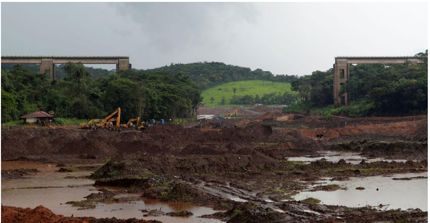
Vale's tailings dam in Brumadinho
